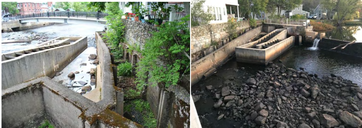
In-use and Abandoned Fishways Views Downstream (left) and Upstream (right)
