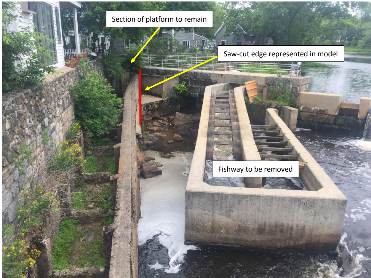
Figure 3-3. Modeled limits of dam removal on river right
