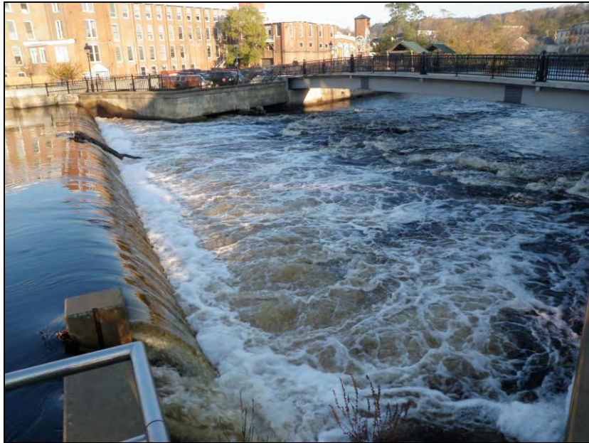
Figure 4a. The Ipswich Mills Dam is a run-of-the-river mill dam formerly used to power the nearby mills. (Horsley Witten Group, November 2011)
