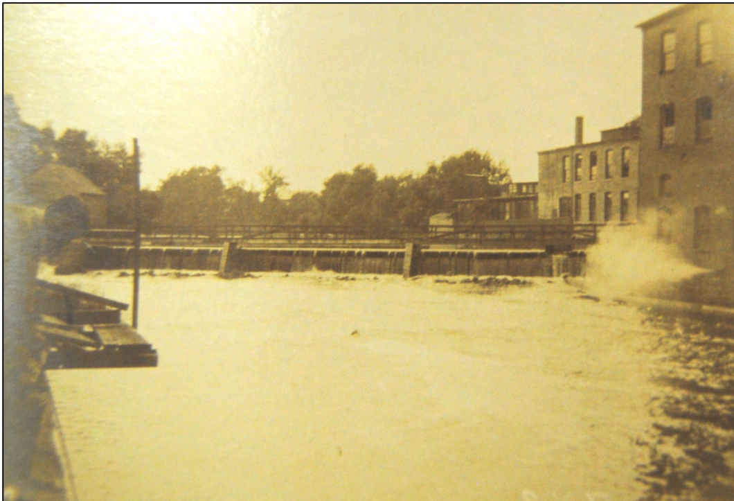
Figure 3. Ca. 1896 photograph of the Ipswich Mills Dam, looking south (upstream) towards dam (source: Courtesy Ipswich Public Library, Ipswich, MA).
