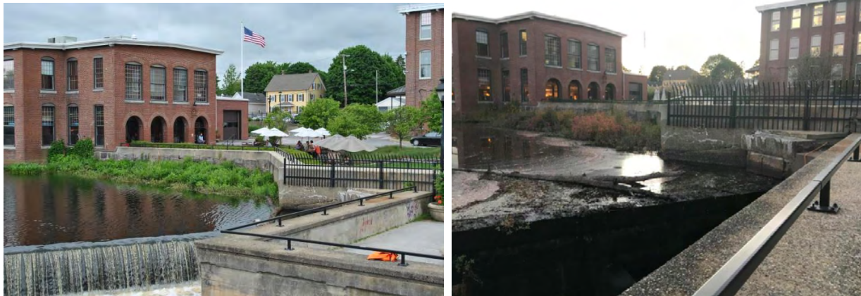
EBSCO Retaining Wall River Left Far-field View (left) and Close-up (right)
