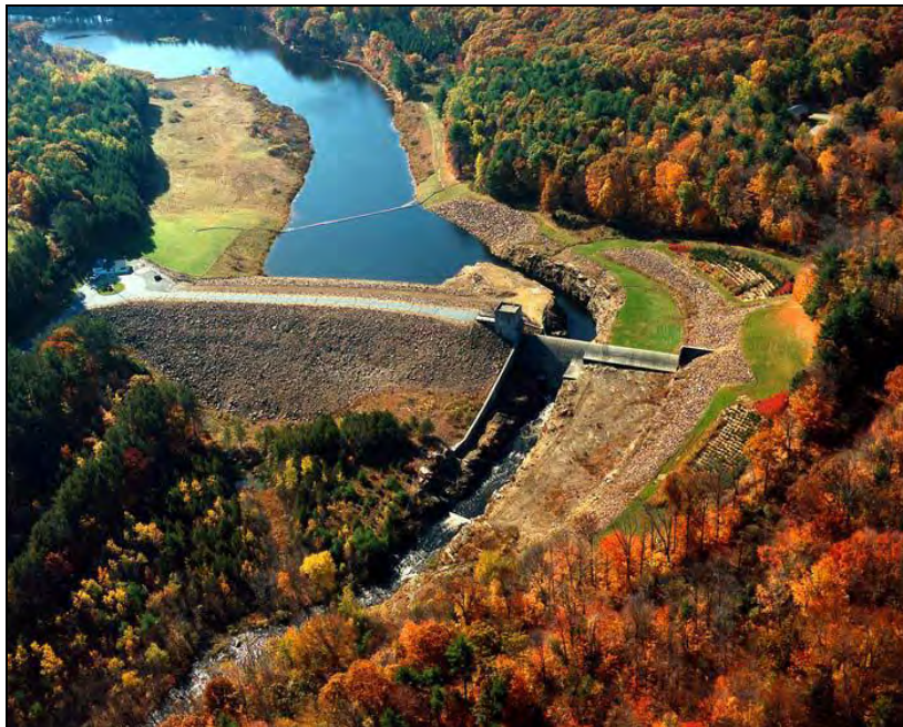
Figure 4b. The Westville Lake Flood Control Dam on the Quinnebaug River in Southbridge, MA serves to control flooding to downstream areas. This dam serves an entirely different purpose than the Ipswich mills Dam. (US Army Corps of Engineers)
