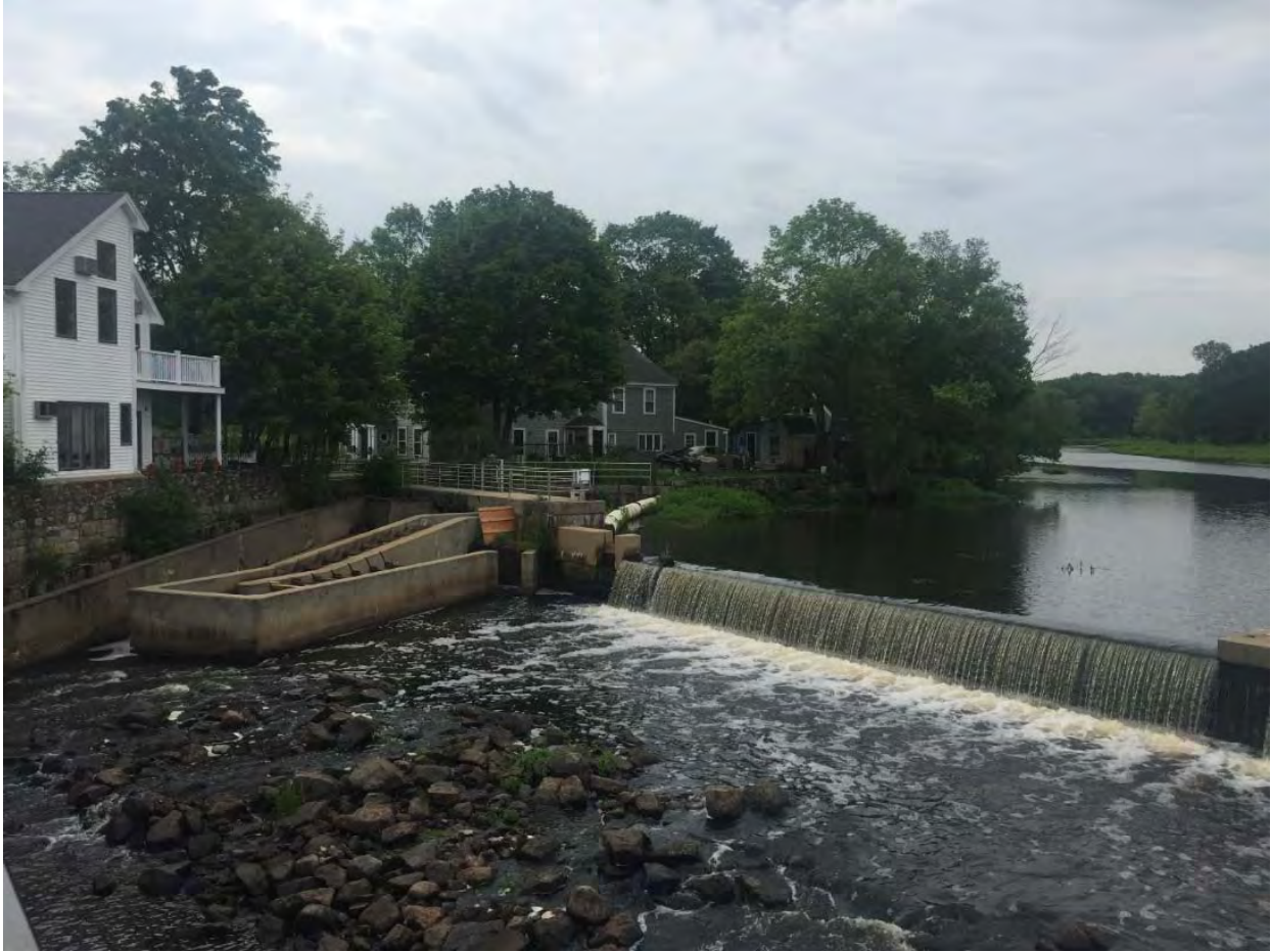
Figure 1. Ipswich Mills Dam
