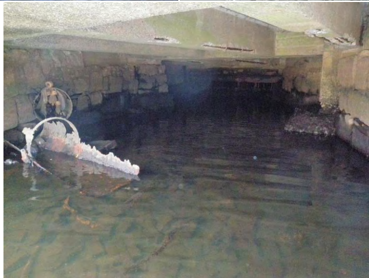
Pedestrian Platform Support Piers Far-field (left), Close-up (right), and Underneath (bottom)
