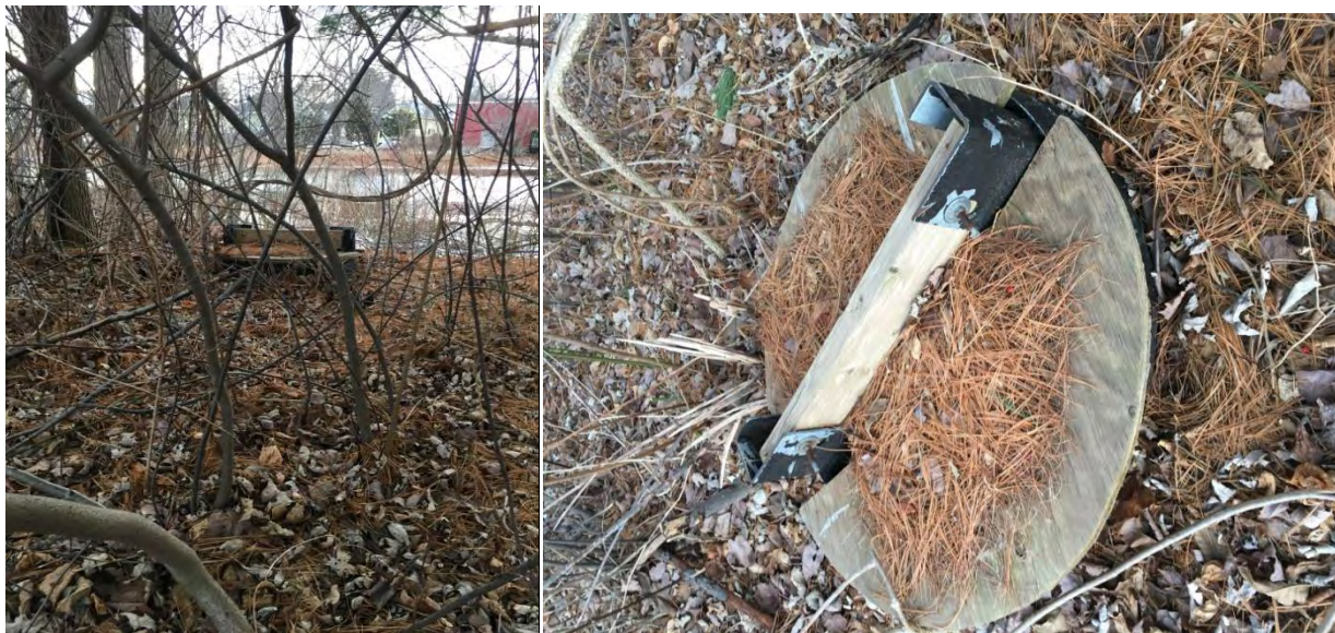
Sally Pond Outlet Control Structure Far-field View (left) and Close-up (right)
