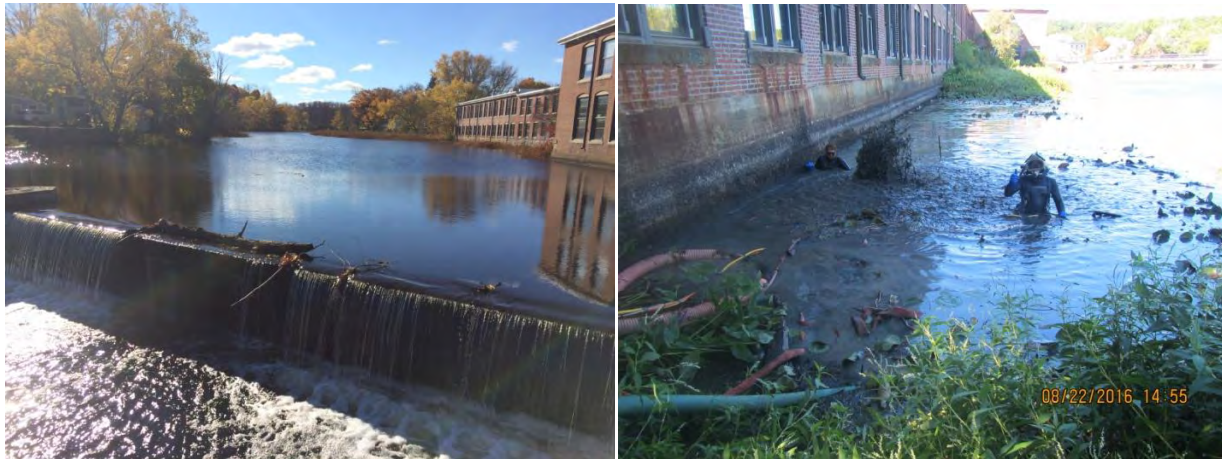
EBSCO Foundation River Left Far-field View (left) and Close-up (right)
