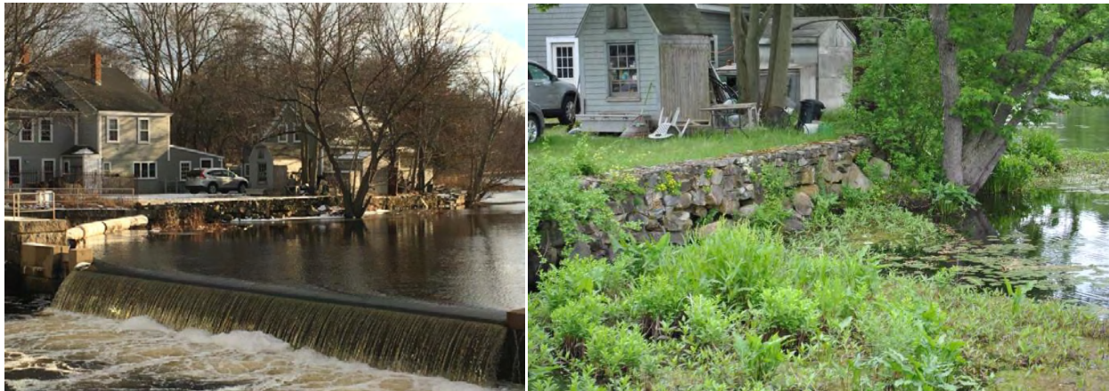
Stone Retaining Wall River Right Far-field View (left) and Close-up (right)
